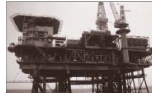
The Chirag-I oil platform, the first development of the Azeri-Chirag-Guneshli oilfields (G Ruschendorf / Rapho / Network)
